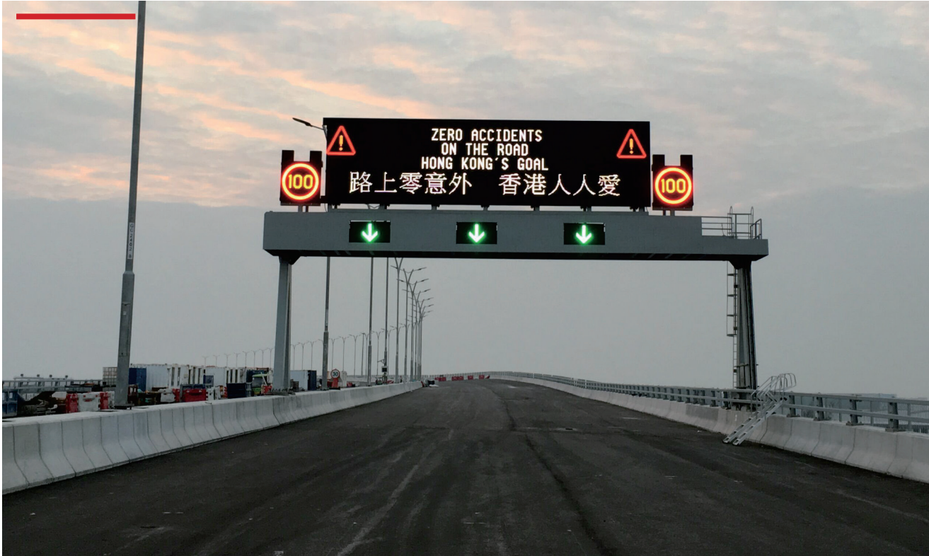
Hong Kong-Zhuhai-Macau Bridge, Hong Kong·China
